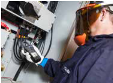
Analyze Power-related Issues
